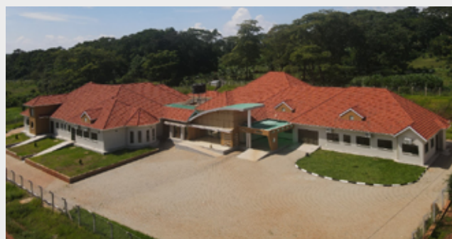
Fig 2. newly constructed multipurpose laboratory to increase NaCORI's capacity for technology development.
